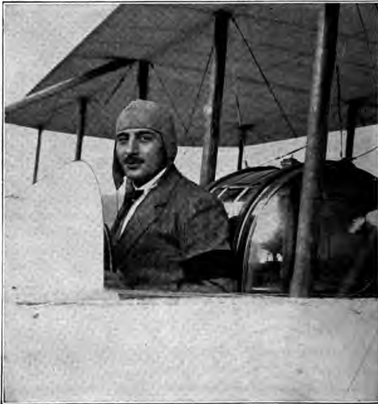
Fig. 8. Close View of Tabuteau Showing Immense Gasoline Supply Tank
